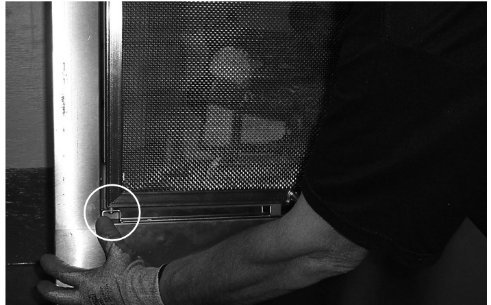
Figure 8 Push Lower Bracket into Place
