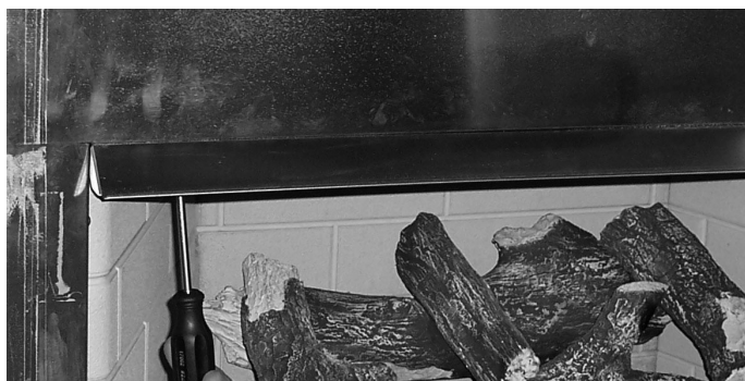
Figure 3 Remove 3 Screws
