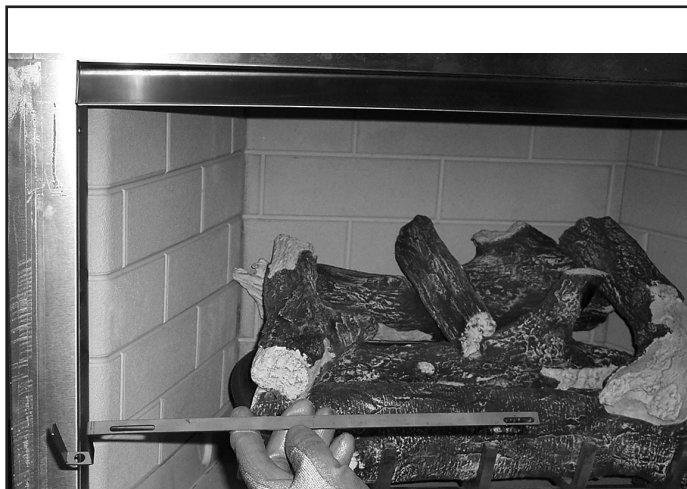
Figure 4 Install Upper Left Bracket
