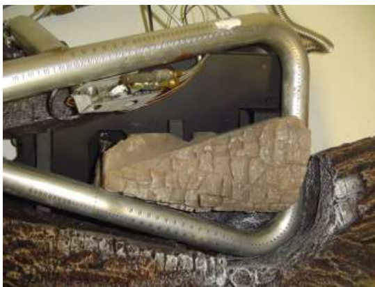
Figure 27A - Installing Charred Log Top View
