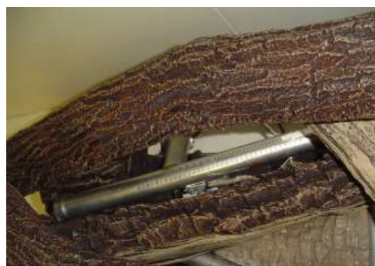
Figure 31A - Installing Back Top Log, Top View
