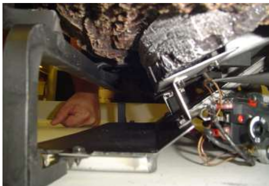
Figure 24C - Installing Right Front Log, Side View
