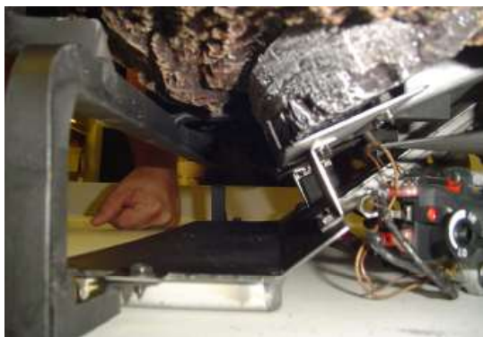
Figure 22C - Installing Right Front Log, Side View
