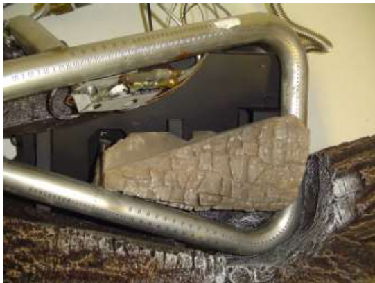
Figure 25A - Installing Charred Log Top View
