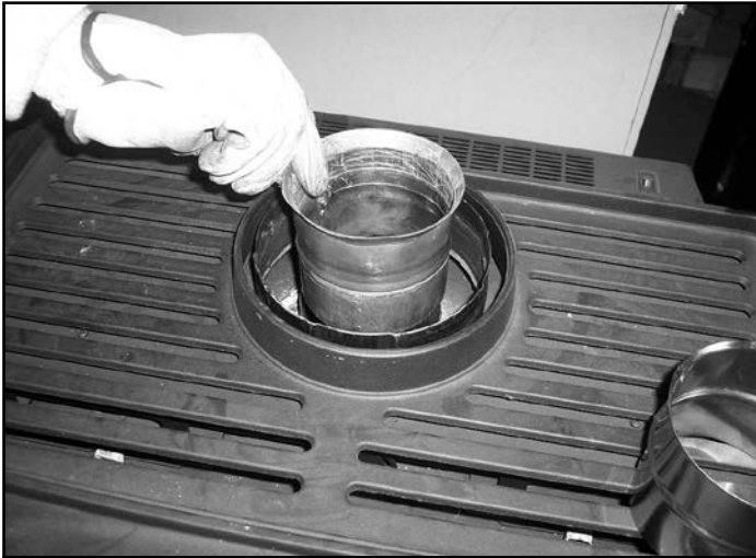
Figure 10 Remove SL-D Adapter
