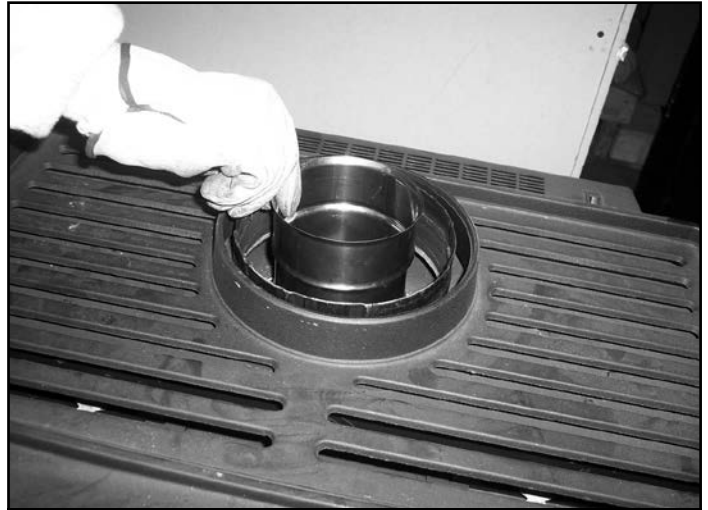
Figure 11 Install SLP-SAM Adapter
