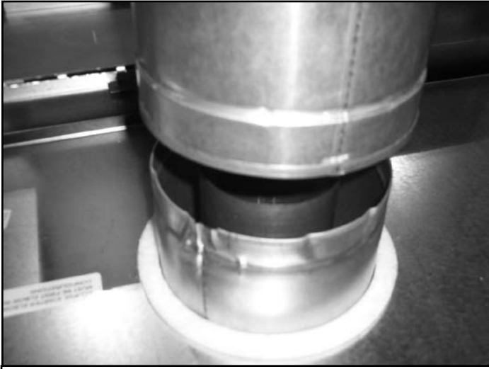
Figure 5 SLP Pipe onto SL-D Collar
