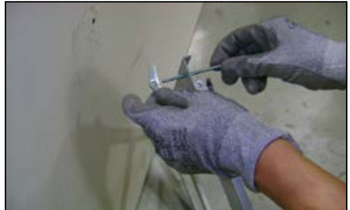
Figure 2 Toggle Bolt Installation through Mounting Bracket
