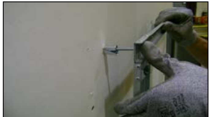
Figure 3 Installing Anchors in Hollow Wall
