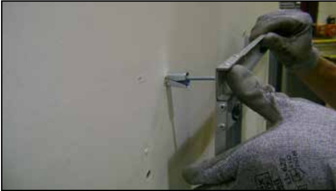
Figure 4.6 Installing Anchors in Hollow Wall
