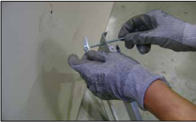
Figure 4.5 Toggle Bolt Installation through Mounting Bracket
