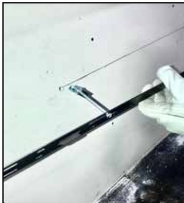
Figure 4.4 Toggle Bolt Installation through Mounting Bracket
