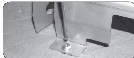
Fig. 16-2 Fasten hammer screws
