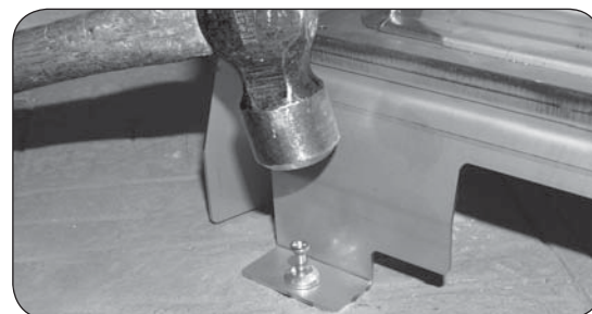
Fig. 16-3 Install hammer screws
