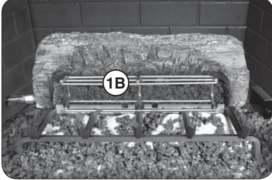
Place the radiant booster grid as shown. The grid should be slid back on the burner up against the rear log. The ember stop has notches to properly align the grid in place.
