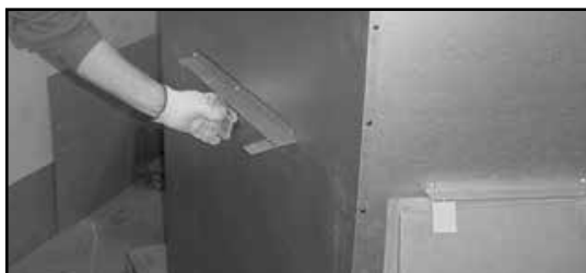
Figure 3.6 Bending Refractory Shipping Tabs Back Down
