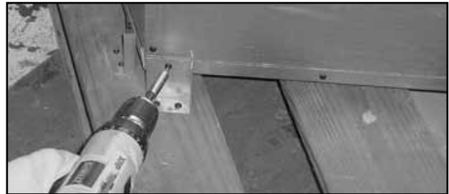
Figure 3.10 Removing Shipping Brackets
