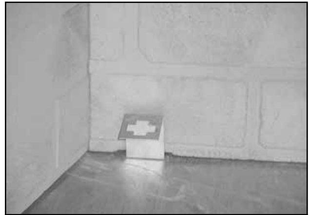
Figure 8.8 Grate Retaining Bracket in Place
