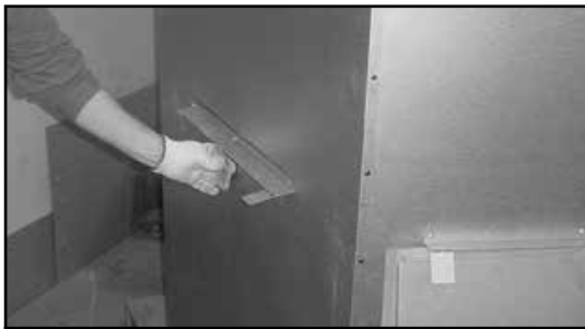
Figure 3.6 Bend Refractory Brackets Back Down
