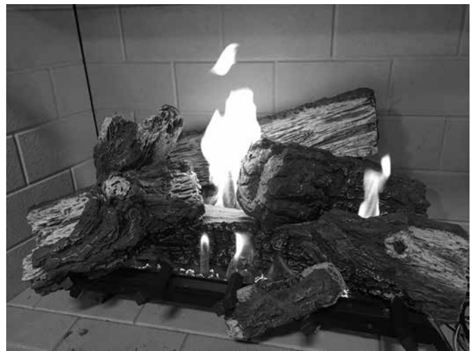
Figure 6.13 - Correct Appearance of Rear Flames
