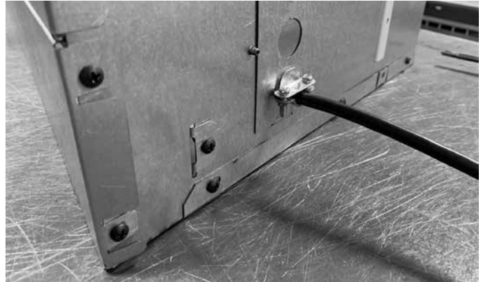
Figure 5.2 Reattaching Junction Box Cover
