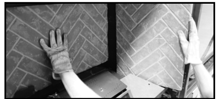
Figure 11.3 Install Side Refractory Panel (Right Side Shown)
