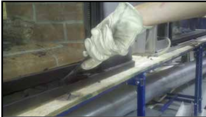
Figure 11.3. Inserting Glass Clip Tool
