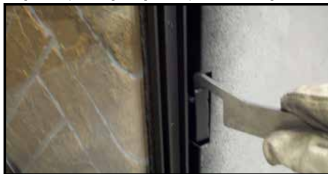
Figure 11.7. Securing Side Glass Clips
