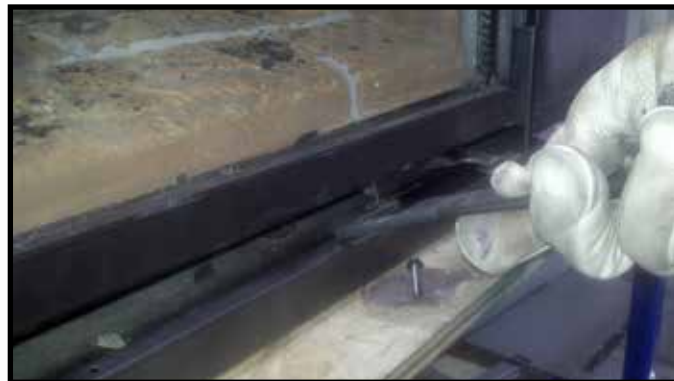
Figure 11.2. Glass Clip Tool Location
