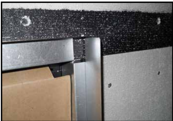
Figure 10.5 Finishing Template Bends
