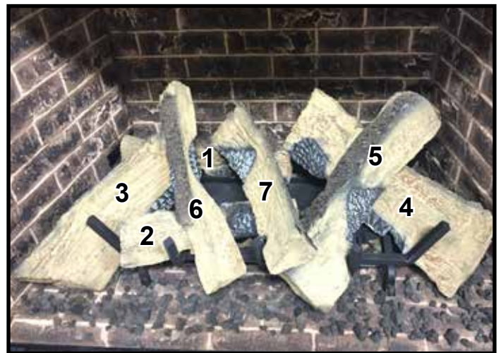
Figure 16. Log Set Installed
