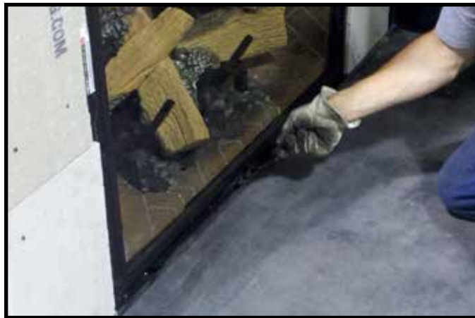
Figure 11.8. Securing Bottom Glass Clips
