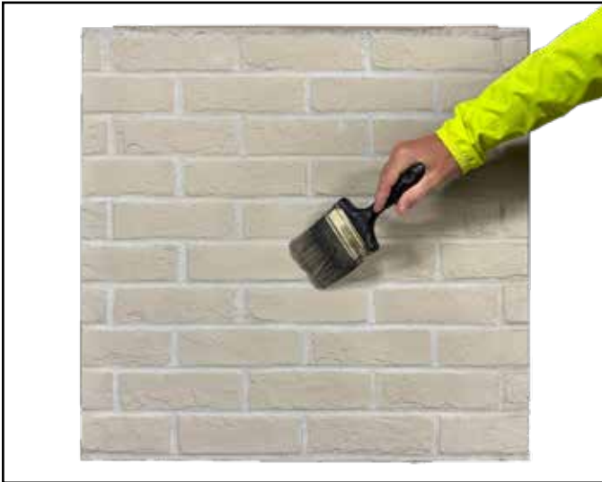
Figure 7 Clean Refractory Panel
