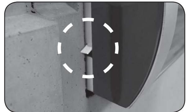
**Fig. 19-1** Tab may interfere when sliding in unit
