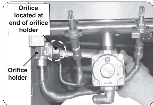
**Fig. 24-3 Orifice location**
