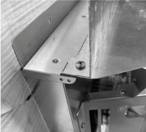
6. Seal seams, corners, and cap to siding using silicone or polyurethane caulk to prevent leaks around cap base.
