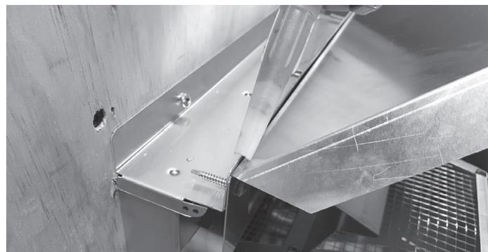
5. Apply bead of high temperature silicone on bottom surface of TRAP-VSS. Position the TRAP-VSS onto cap as shown and attach with (3) screws provided. Clean excess silicone as needed.
