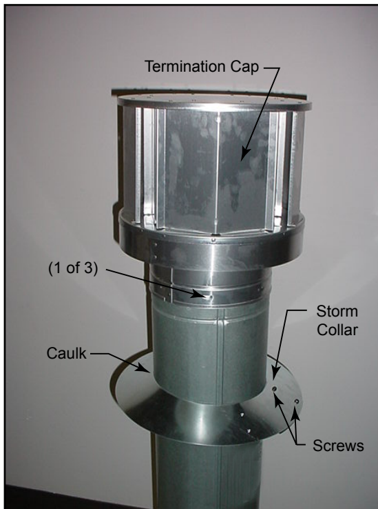
Figure 26 Secure with Screws
