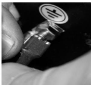
8. Connect gas inlet fitting to mains gas supply in accordance with local gas installation code and gas supply installation section of manual. Leak test with soapy water.
