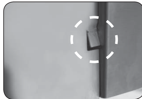
Fig. 13-2 Tab slightly bent in for clearance
