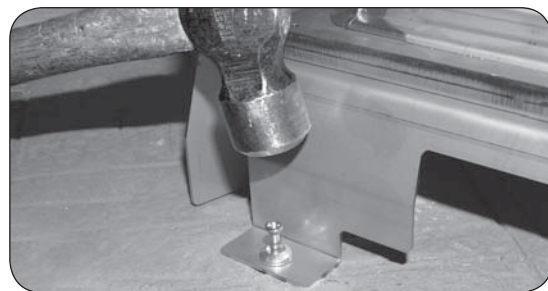
Fig. 16-2 Install hammer screws
