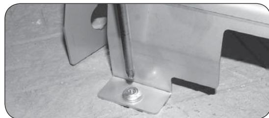
Fig. 16-3 Fasten hammer screws
