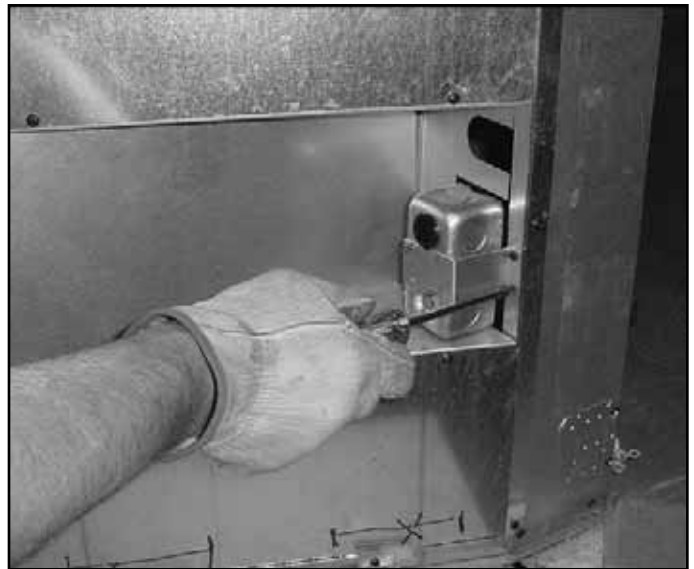
Figure 13.2 Remove Two Screws From Bracket
