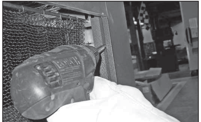
Figure 15.15 Install Refractory Shields
