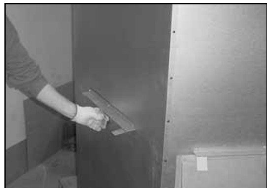
Figure 7.2 Bending Refractory Shipping Tabs Back Down
