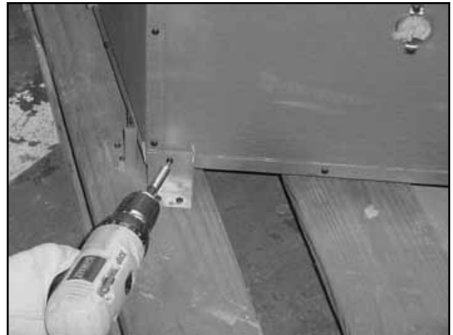
Figure 7.7 Removing Shipping Brackets
