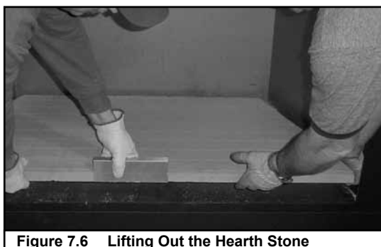
Figure 7.6 Lifting Out the Hearth Stone
