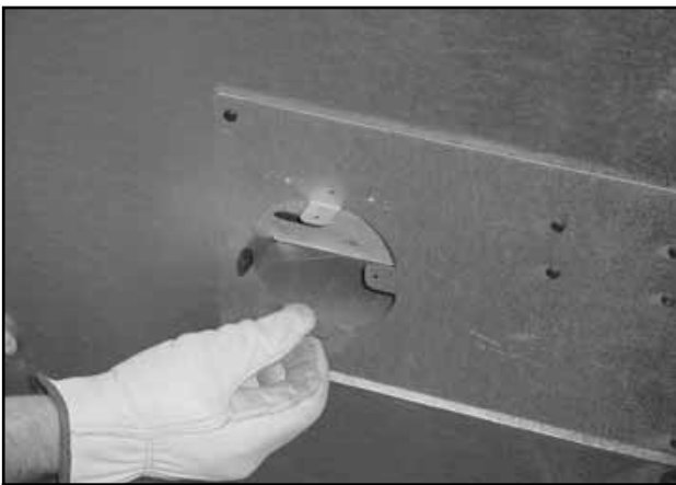
Figure 7.20 Bending Tabs on Outside Air Kit Collar
