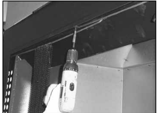
Figure 7.3 Remove Screen Rods
