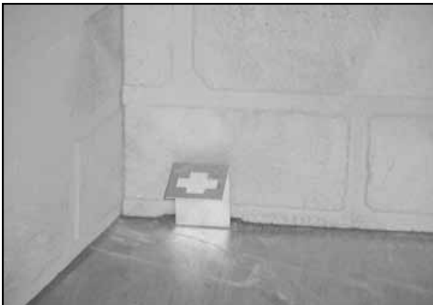
Figure 7.16 Grate Retaining Bracket in Place
