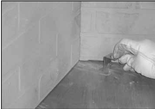
Figure 7.15 Slide Grate Retaining Bracket into Notch
