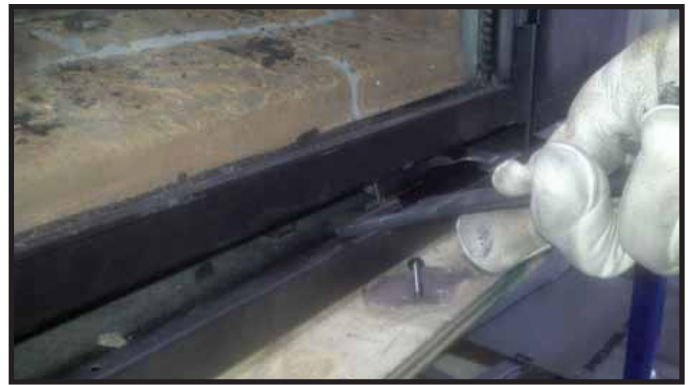
Figure 14.7. Glass Clip Tool Location
