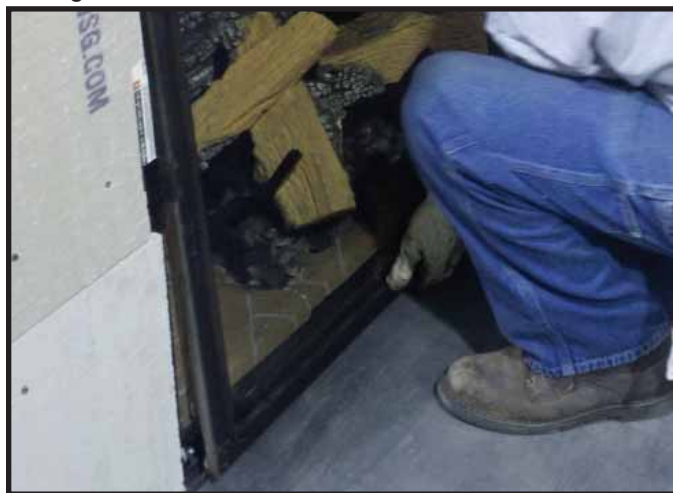
Figure 14.11. Installing Glass
