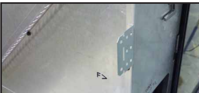
Figure 9.3 Nailing Tab Bent Out for Installation
