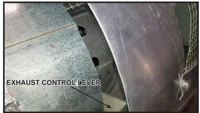
Figure 7.10 PVK-80 Control Lever Adjustment - Open
