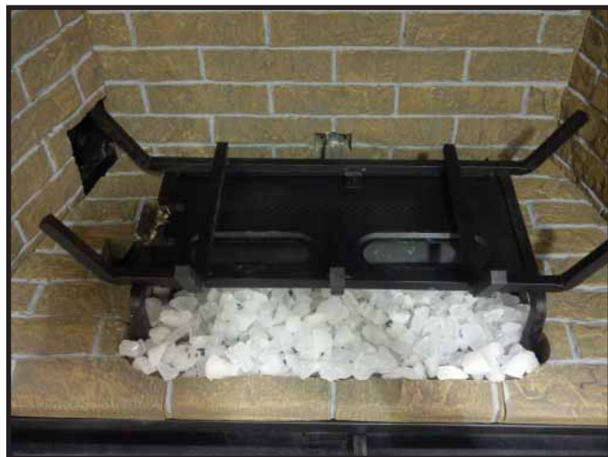
Figure 14.2. Ember Glass Area Covered with Teco-Sil
