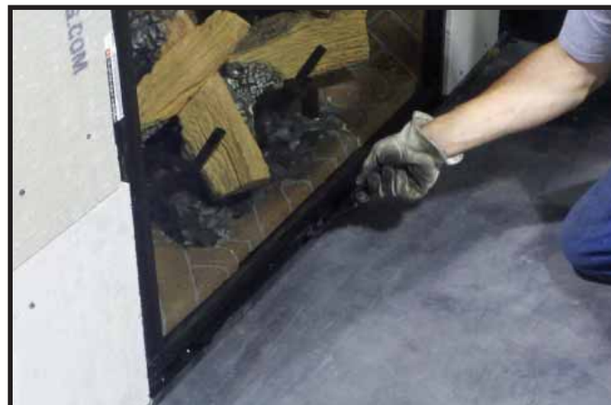
Figure 14.13. Securing Bottom Glass Clips
