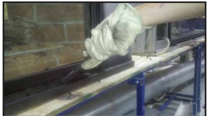
Figure 14.8. Inserting Glass Clip Tool
