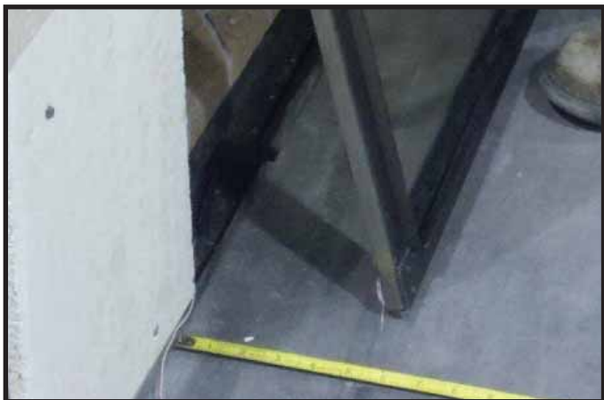
Figure 14.9 Positioning Glass
