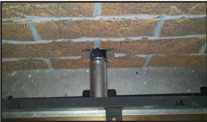
Figure 14.14 Air Shutter
