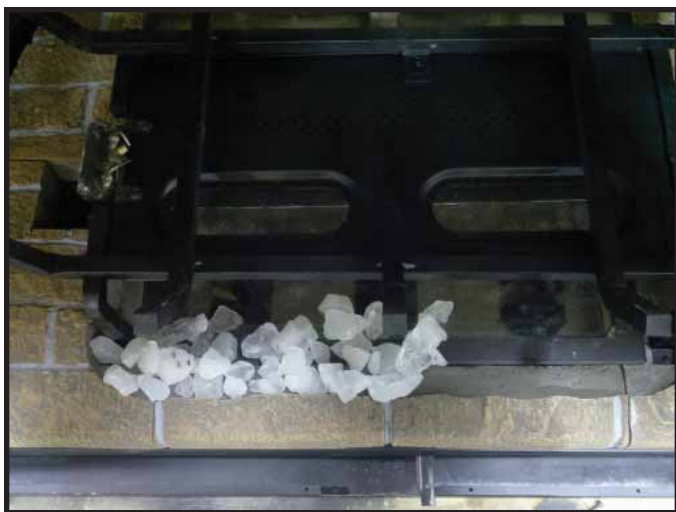
Figure 14.1. Install Teco-Sil
