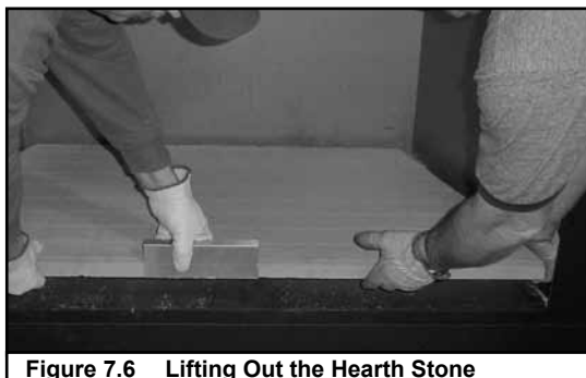
Figure 7.6 Lifting Out the Hearth Stone
