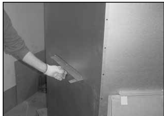
Figure 7.2 Bending Refractory Shipping Tabs Back Down
