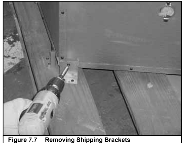
Figure 7.7 Removing Shipping Brackets
