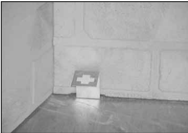
Figure 7.16 Grate Retaining Bracket in Place
