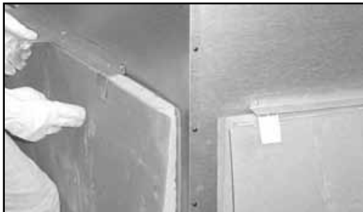
Figure 7.1 Unpack Back Refractory
