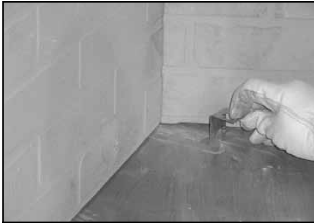
Figure 7.15 Slide Grate Retaining Bracket into Notch
