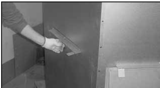
Figure 7.2 Bend Refractory Brackets Back Down
