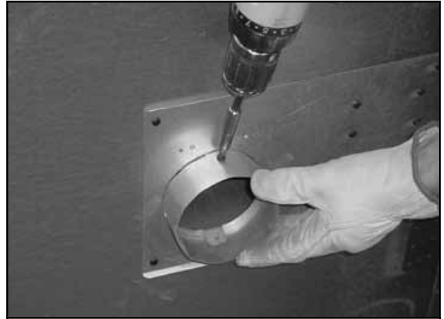
Figure 7.21 Attaching Outside Air Kit Collar
