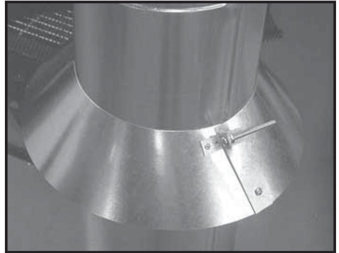
Figure 8.17 Assembling the Storm Collar Around the Pipe
