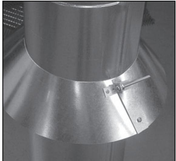
Figure 4.6 Assembling the Storm Collar Around the Pipe
