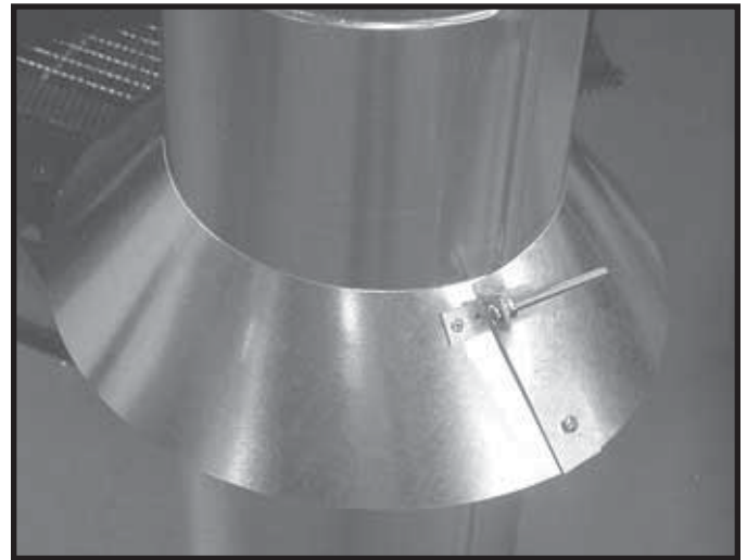
Figure 8.17 Assembling the Storm Collar Around the Pipe
