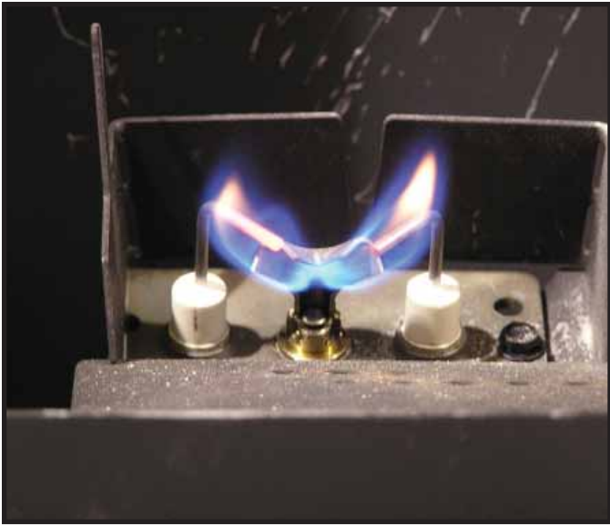
Figure 3.1 IPI Pilot Flame Patterns
