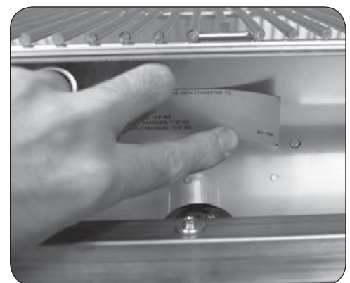
Fig. 4-3 Apply the conversion label
