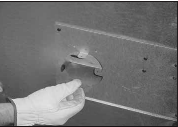
Figure 3.18 Bending Tabs on Outside Air Kit Collar
