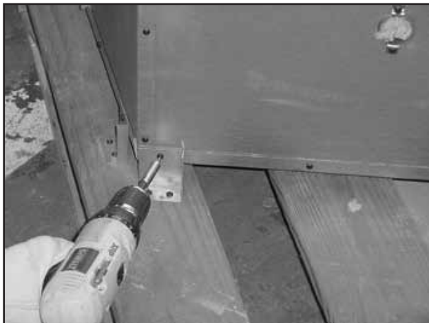
Figure 3.6 Removing Shipping Brackets
