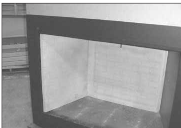
Figure 8.6 Side Refractory Installed
