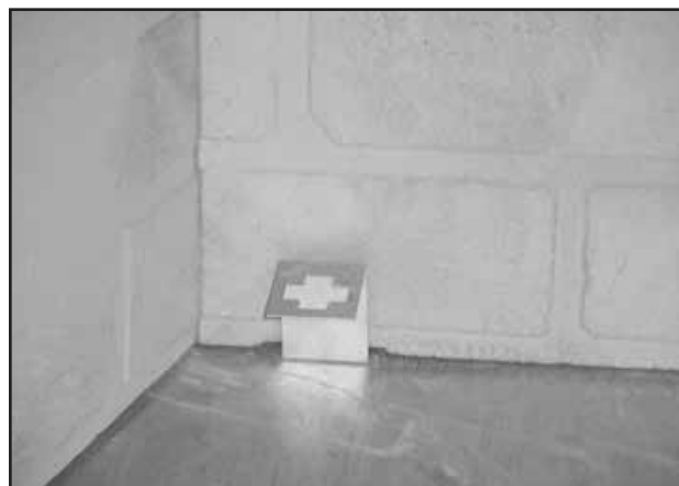
Figure 8.8 Grate Retaining Bracket in Place
