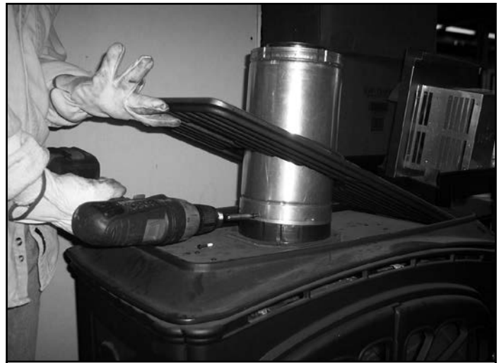
Figure 7 Fasten SLP Vent to Stove
