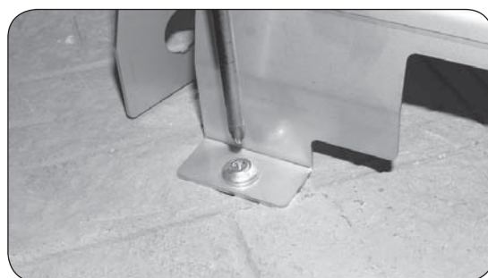
Fig. 14-4 Fastening hammer screws
