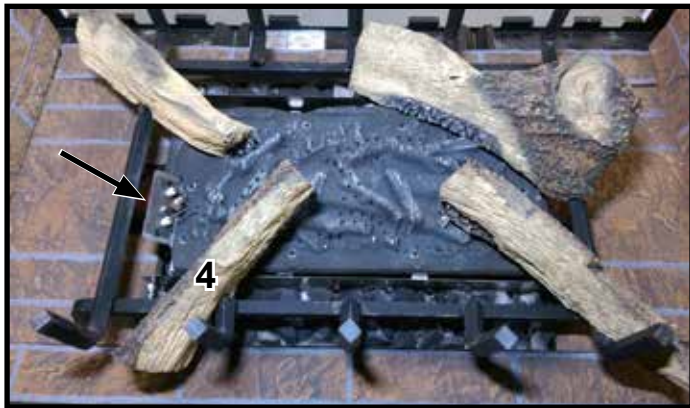
Figure 10. Log #4 from front showing grate tine groove.
