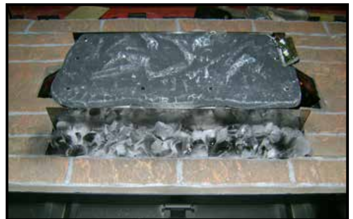
Figure 11.16 Finished Ember Bed
