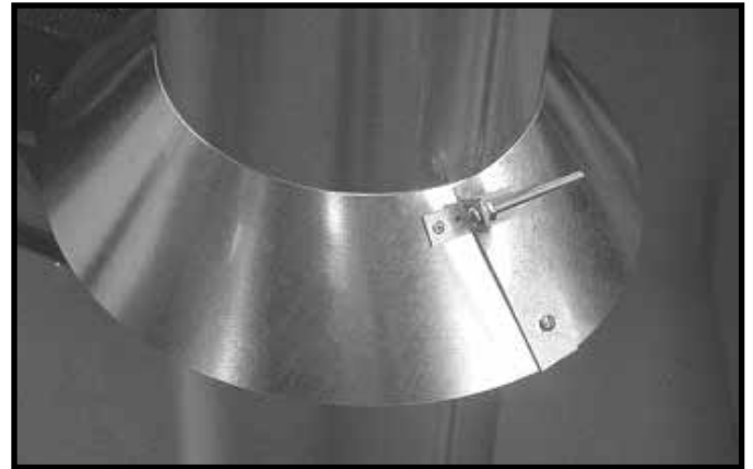
Figure 7.12 Insert Bolt into Brackets
