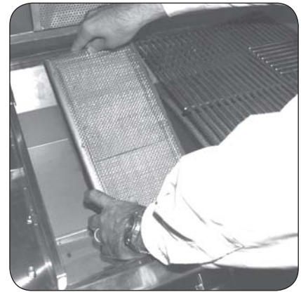
Fig. 4-2 Install new burner
