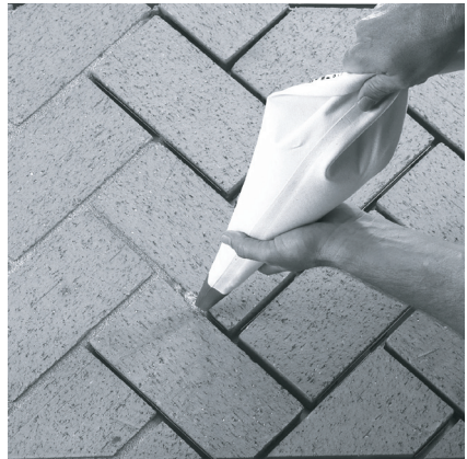
Figure 4 - Grouting
