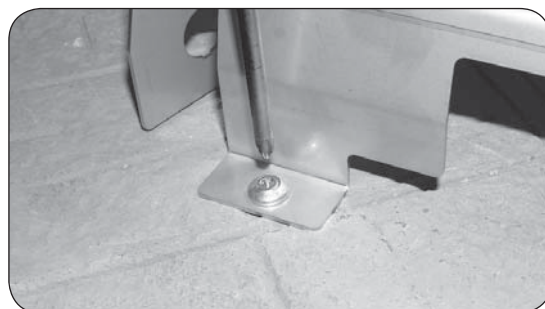
Fig. 14-4 Fastening hammer screws
