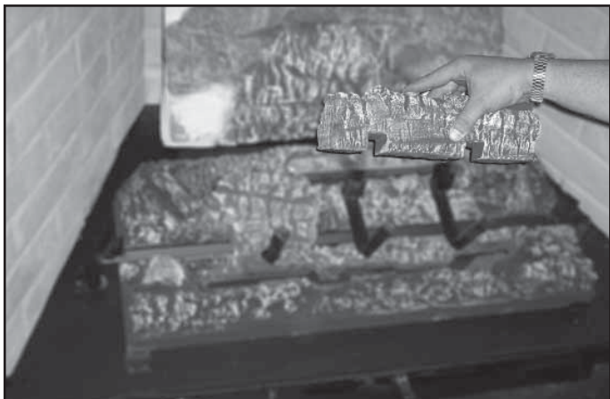
Figure 15.12 Positioning Right Front Log
