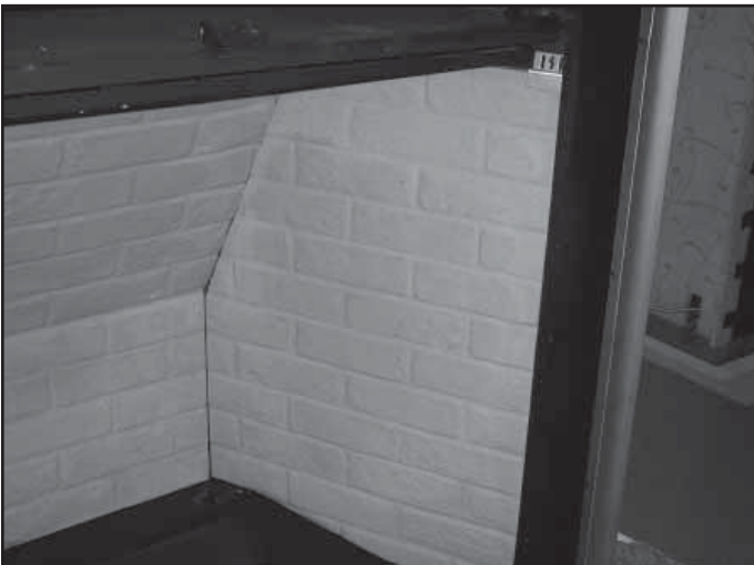
Figure 15.5 Install Right Side Refractory
