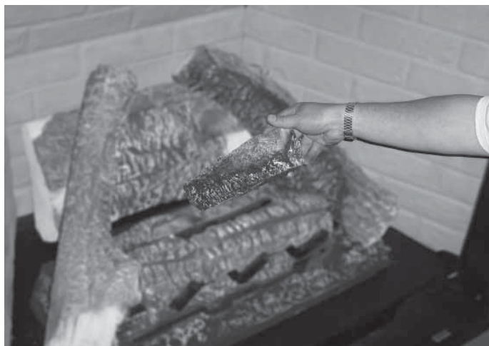
Figure 15.15 Positioning Right Middle Log
