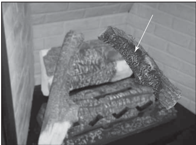
Figure 15.14 Positioning Right Log
