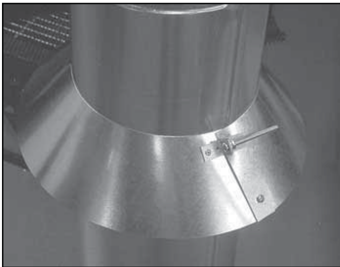
Figure 10.14 Assembling the Storm Collar Around the Pipe
