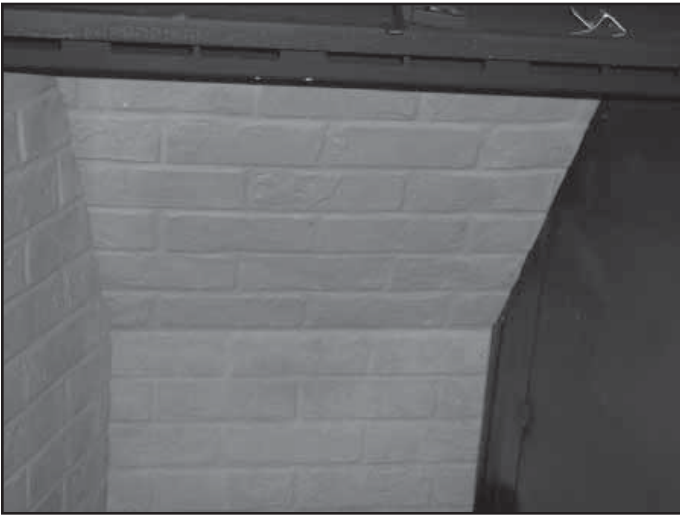
Figure 15.4 Install Upper Back Refractory
