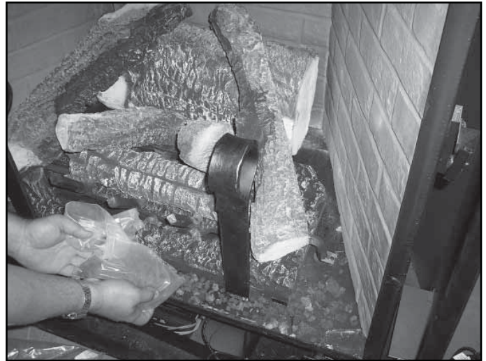
Figure 15.19 Placing Lava Rock
