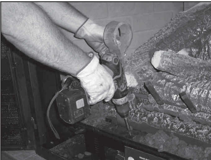
Figure 15.18 Installing Andirons
