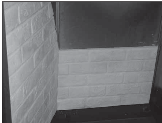
Figure 15.3 Install Lower Back Refractory
