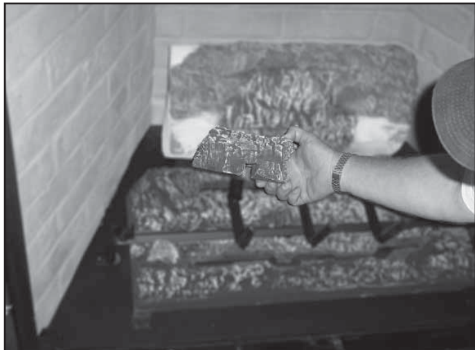
Figure 15.11 Positioning Left Front Log
