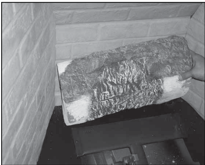
Figure 15.8 Positioning Rear Log
