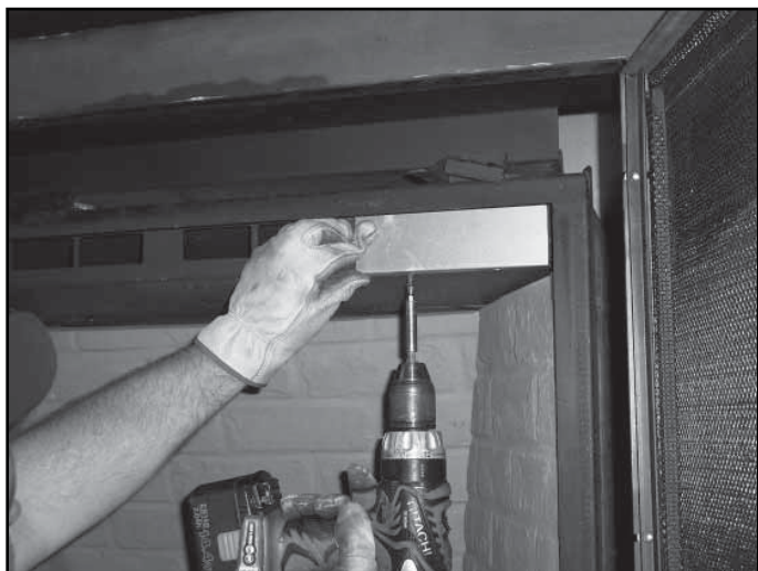
Figure 15.7 Adjust the Vertical Baffle
