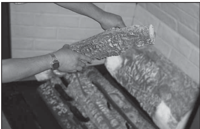
Figure 15.13 Positioning Left Log
