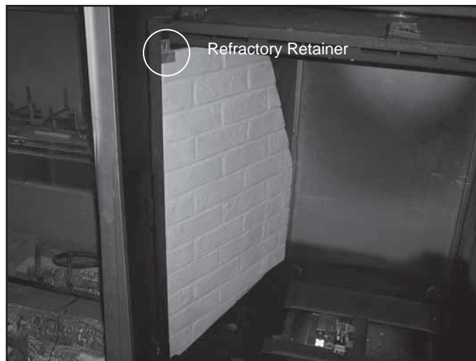
Figure 15.2 Install Left Side Refractory
