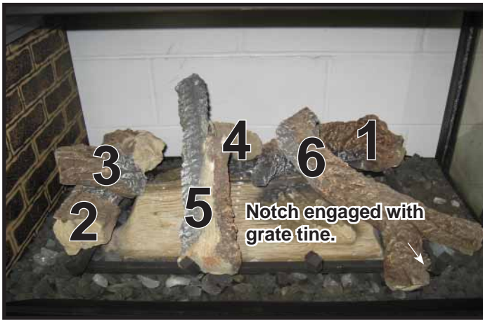
Log Assembly Installed.
