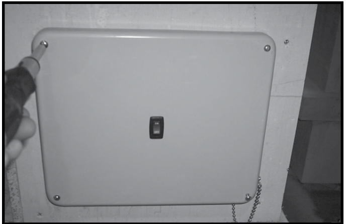
Figure 5.9 Replace Control Cover
