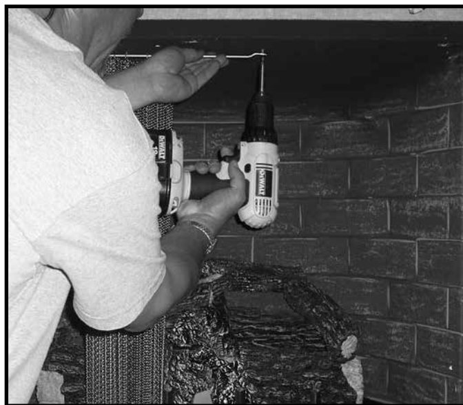
Figure 8.17 Fasten Screen Rod to Firebox Top
