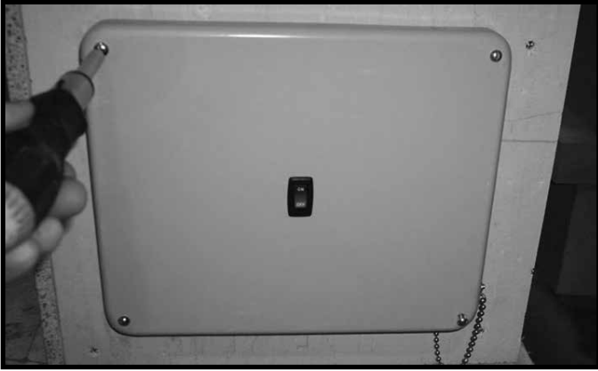
Figure 5.1 Remove Control Cover
