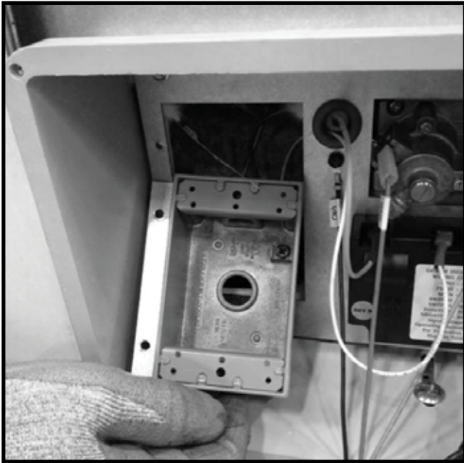
Figure 5.6 Place & Fasten Junction Box
